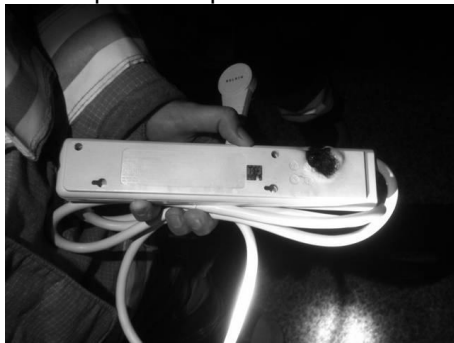
Burned power strip
